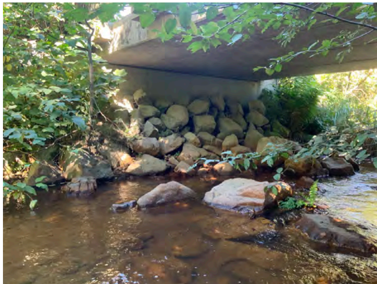
Right Bank Abutment when facing downstream
