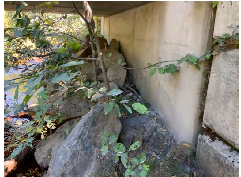
Left Bank Abutment when facing downstream
